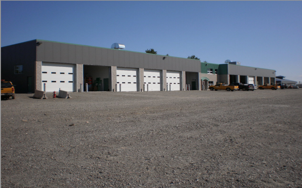
Norbec Panels used instead of tilt up for economic reasons on The Department of Transport District 4 Maintenance Depot
